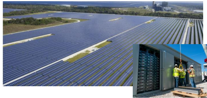
The Manatee Energy Storage Center able to deliver 900 MWh of energy – enough to power 329,000 homes for two hours.
